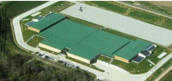
Walmart's Data Center
